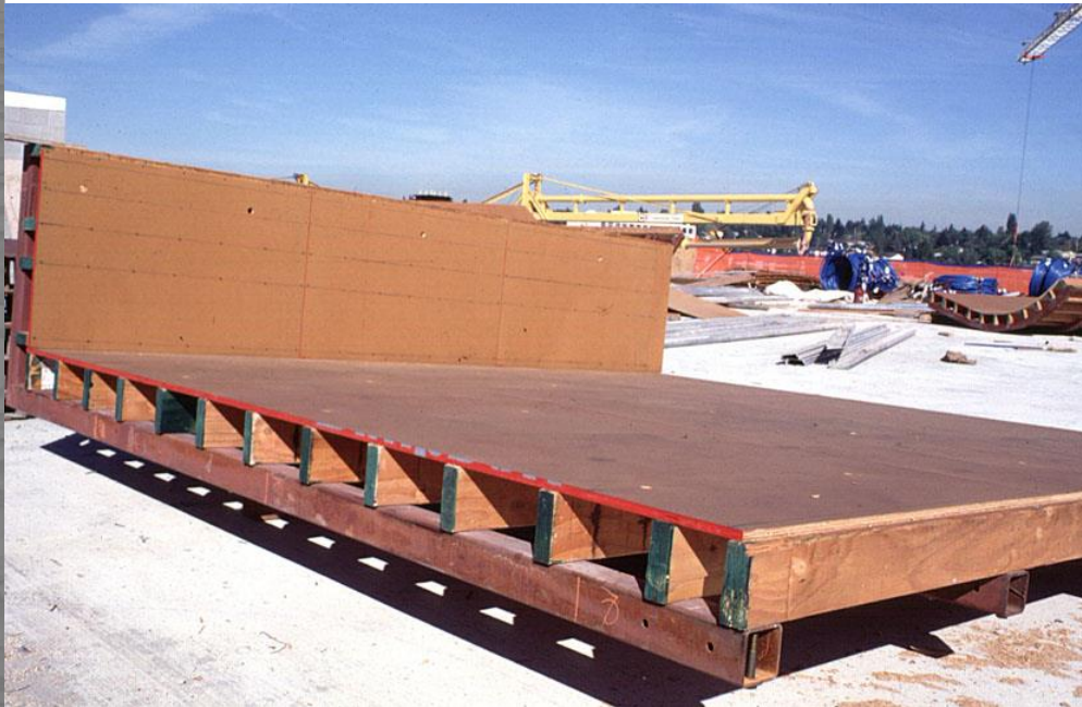
Concrete Forming - MDO
